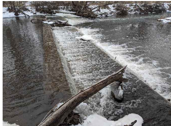
1 G03 EXISTING CONCRETE WEIR
