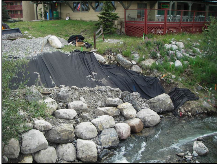
Figure 4.5. Filter fabric installation example
