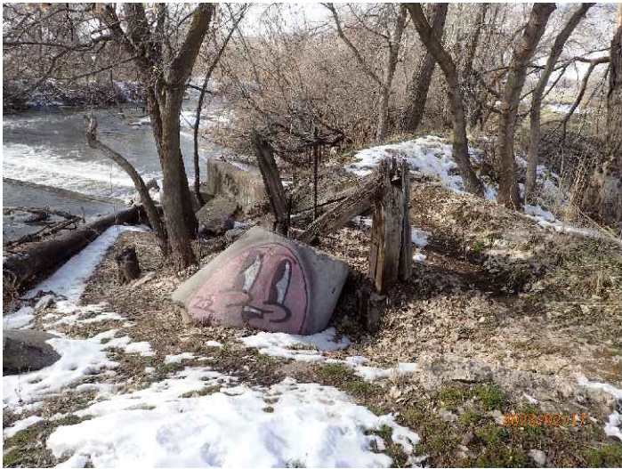
4 G03 EXISTING ABANDONED CONCRETE MANHOLE CAP & ABANDONED HEADGATE
